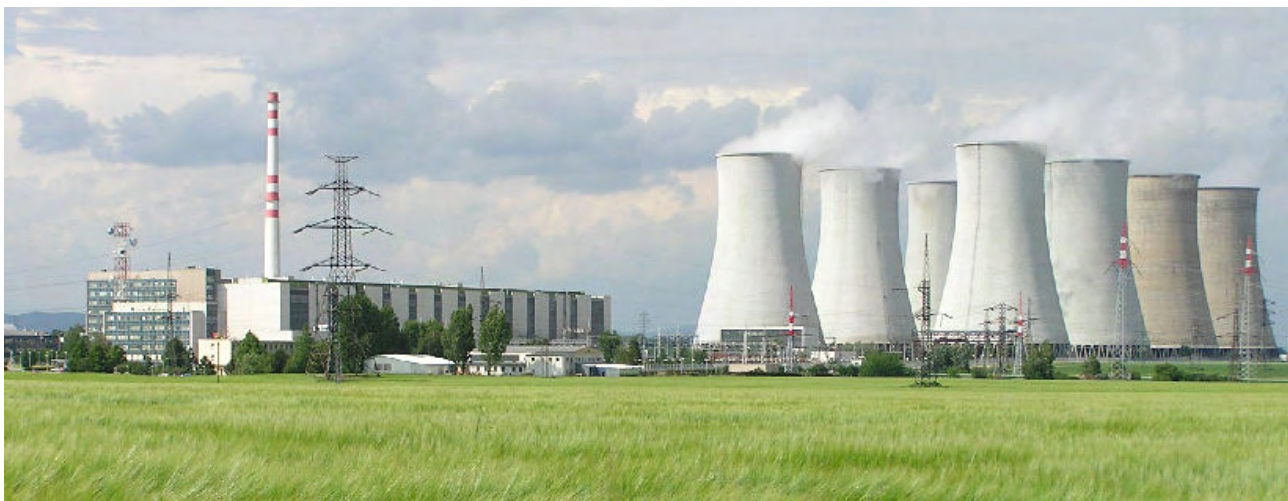
Figure 1: View of V1 NPP from the southeast.
