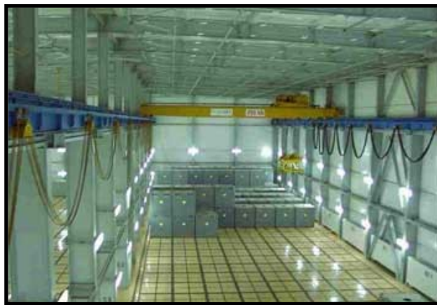
FIGURE 2.2-27 TEMPORARY STORAGE IN THE STORAGE HOUSE FOR STORAGE OF CONDITIONED RAW ON THE SITE OF NPP KOZLODUY
