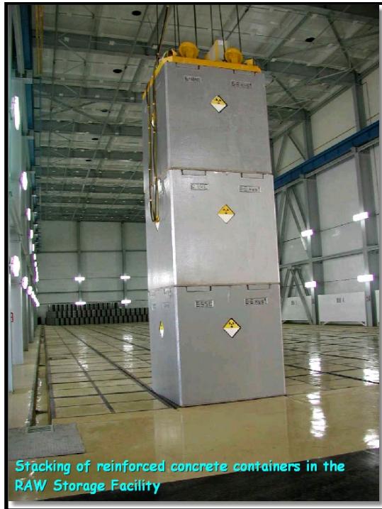
FIGURE 2.2-26 REINFORCED CONCRETE CONTAINERS OF DISPOSAL OF RAW IN NDF
