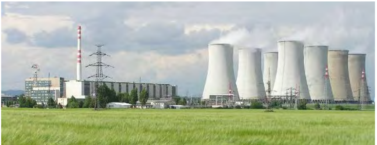
Figure A-2: View of V1 NPP from the southeast.
