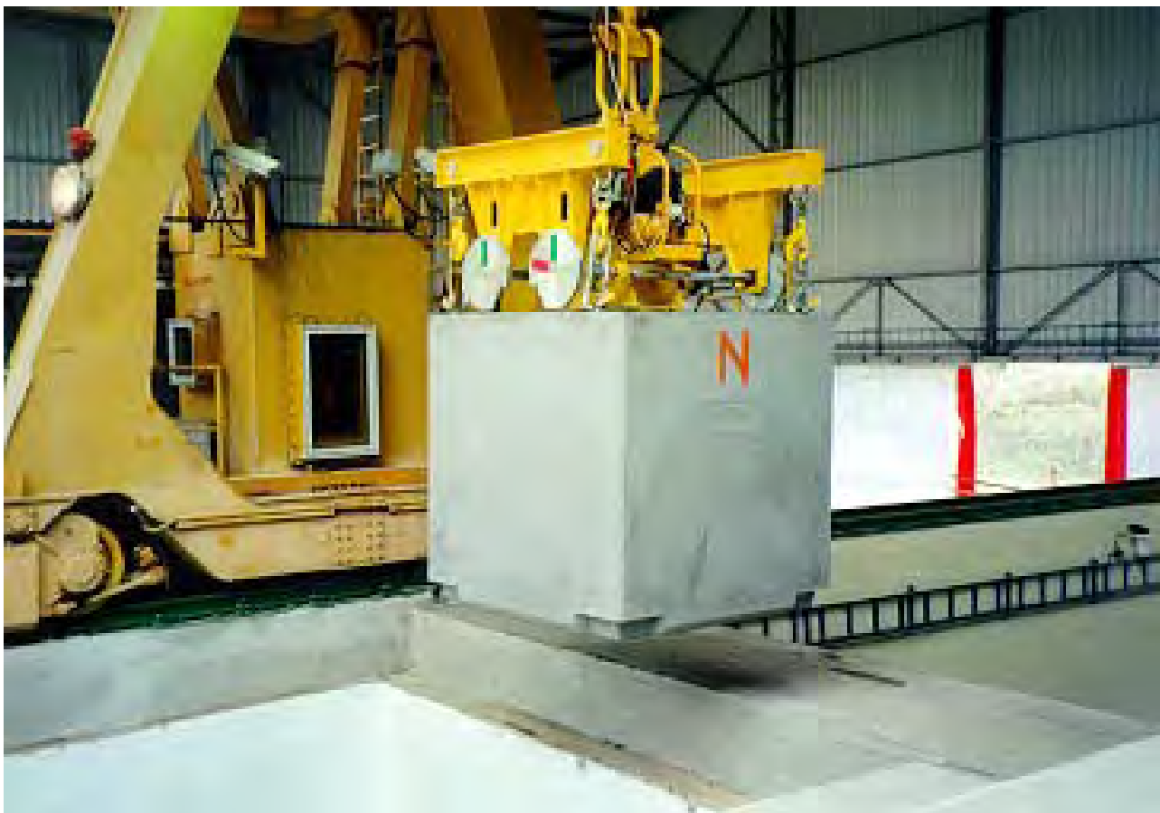
Figure B-4: Insertion of RAW packaged form (FCC) to the storage chamber of near-surface repository in Mochovce
